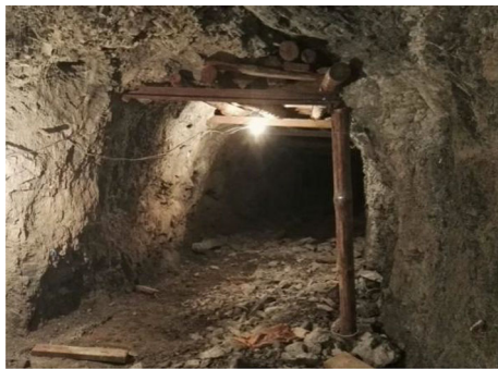
Fig. 2 Failure diagram of roadway side wall blasting
