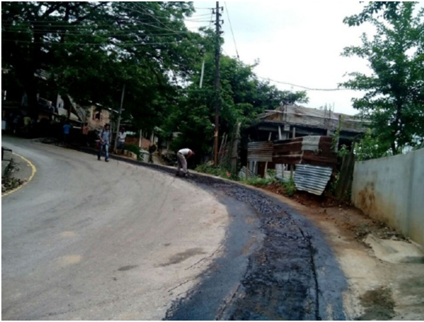
Fig. 7 Road open to traffic
