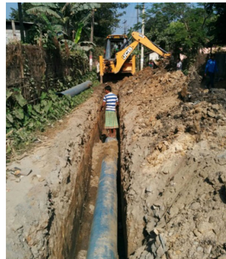
Fig. 6 Removal of debris
