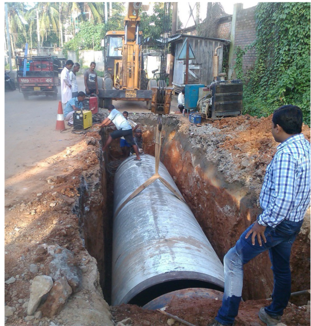
Fig. 3 Laying and jointing of pipes
