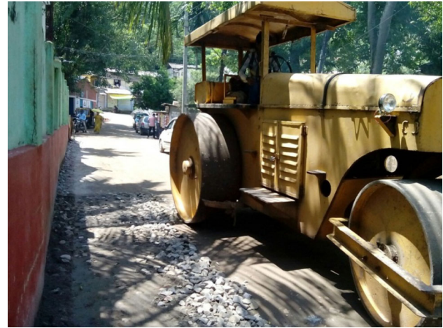
Fig. 5 Stages of road restoration
