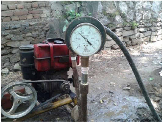
Fig. 4 Hydro testing of pipelines
