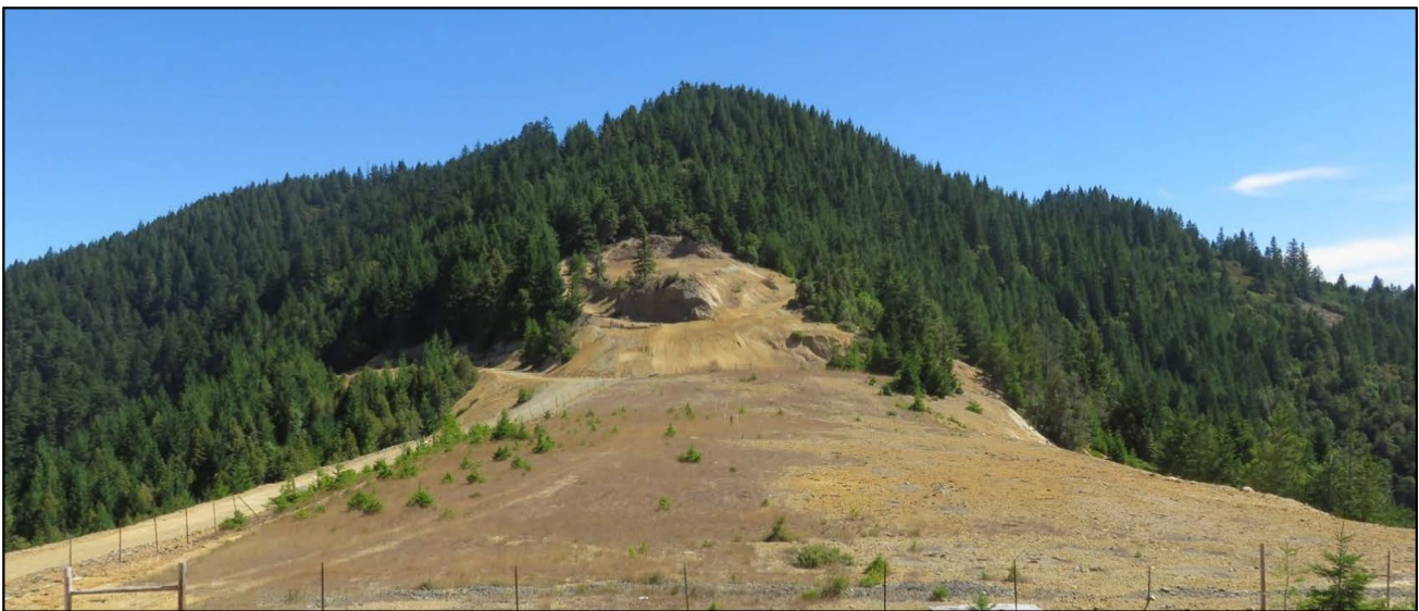
Fig. 1 An eastward view of the aboveground remains at the abandoned Formosa Mine site near Riddle, Oregon, USA. A large encapsulation mound (foreground) was a repository for low-
