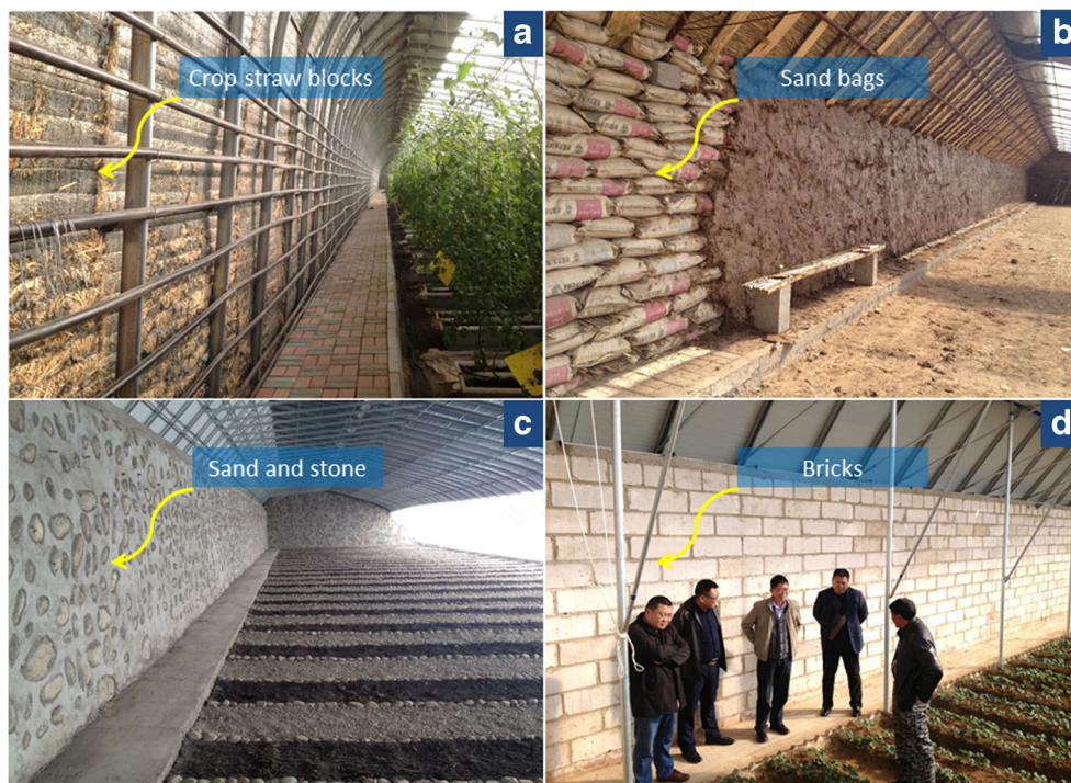
Fig. 7 Locally available materials are used to make the north wall of the cultivation units, including (a) steel-framed and straw-stuffed blocks, (b) sandbags, (c) stone–cement mixture, and (d) common bricks, among others
