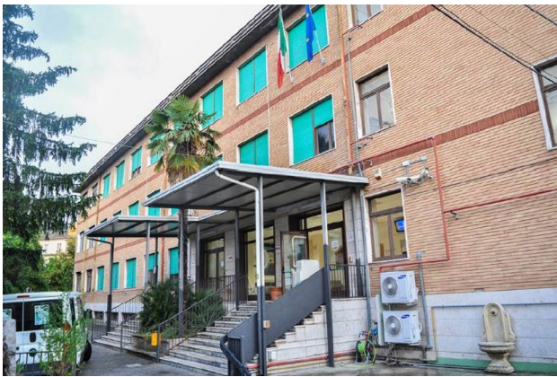
Fig. 1 Building hosting the masonry partition
