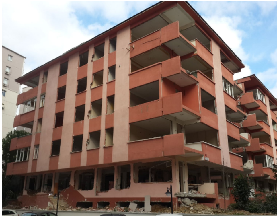
Fig. 1 Studied building with its twin on the right-hand side
