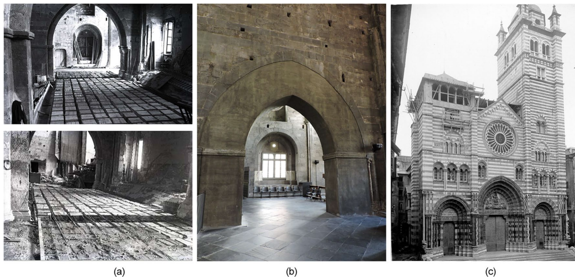
Fig. 2 Past structural interventions realized on the bell tower: (a, b) r.c. slabs and arch realized in 1929 in the matroneum; c demolition of the wall connecting the two towers in 1933
