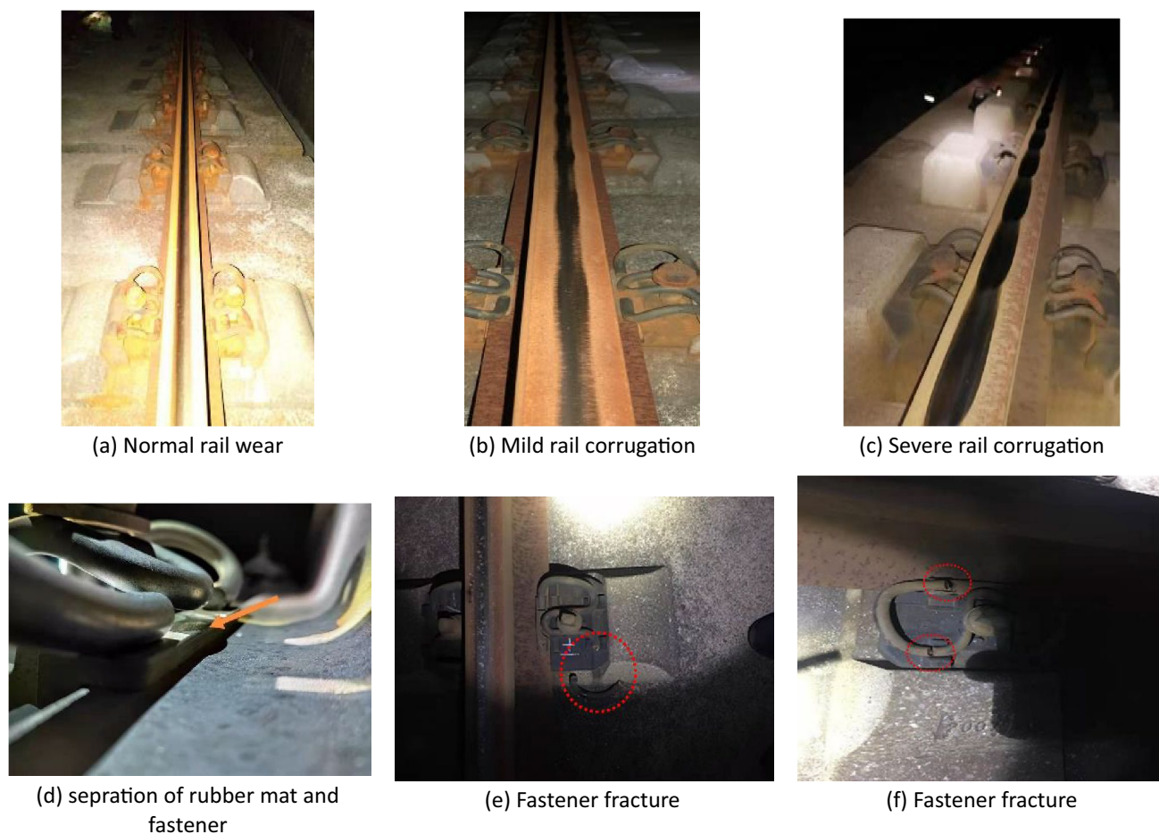
Fig. 1 Three types of rail corrugations and rail running surfaces
