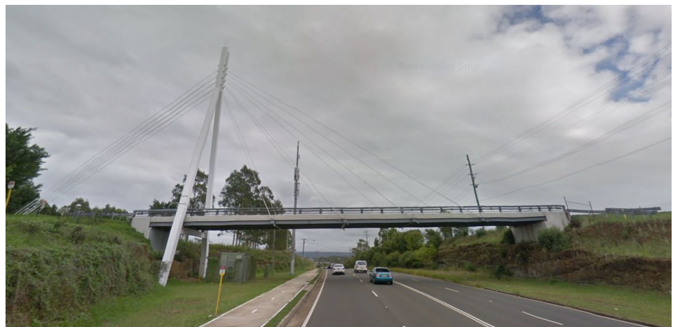
Fig. 3 Side view of the cable-stayed bridge from our first case study, Western Sydney, Australia (source: Google Earth)
