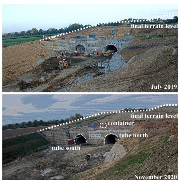
**Fig. 1** East tunnel portal before terrain modeling (July 2019) and after major terrain modeling (November 2020) [10]
