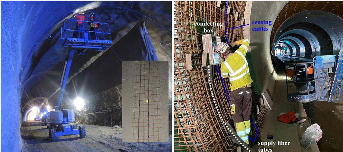
**Fig. 3** Installation of sensing cables along the shotcrete lining [10] (left) and inside the inner tunnel lining (right)
