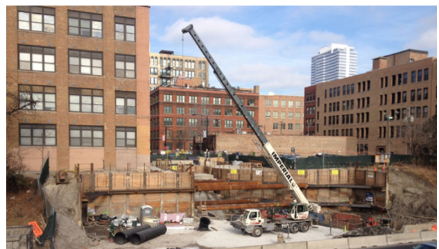
Fig. 10 The historical building at Chicago and excavations adjacent to it [34]
