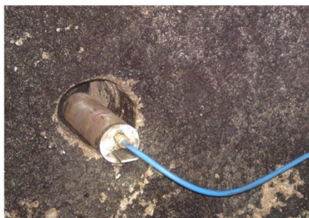
Fig. 5 FBG geophone installed horizontally.
