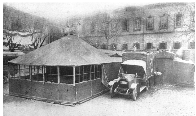
Fig. 1 The core of the Mobile Surgical Hospital “Città di Milano”. The operating cabin-tent, connected with the two preparation tents and sided by the Fiat 15-ter truck that transported it and whose engine, once the cabin was installed, remained connected to the operating tent to provide energy for warming and illumination
