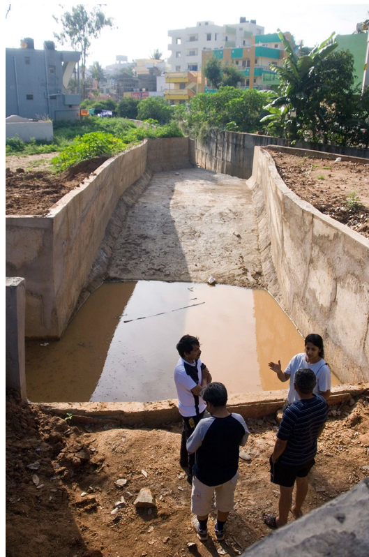
Fig. 5 Members of a lake group inspecting the restoration work done by city authorities to regulate the flow of water from one of the group’s lakes to the one downstream (photo by Johan P. Enqvist)
