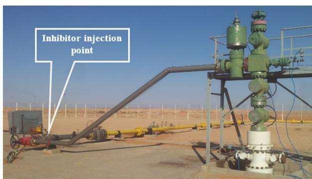
**Fig. 6** Injection point of corrosion inhibitor at the wellhead
