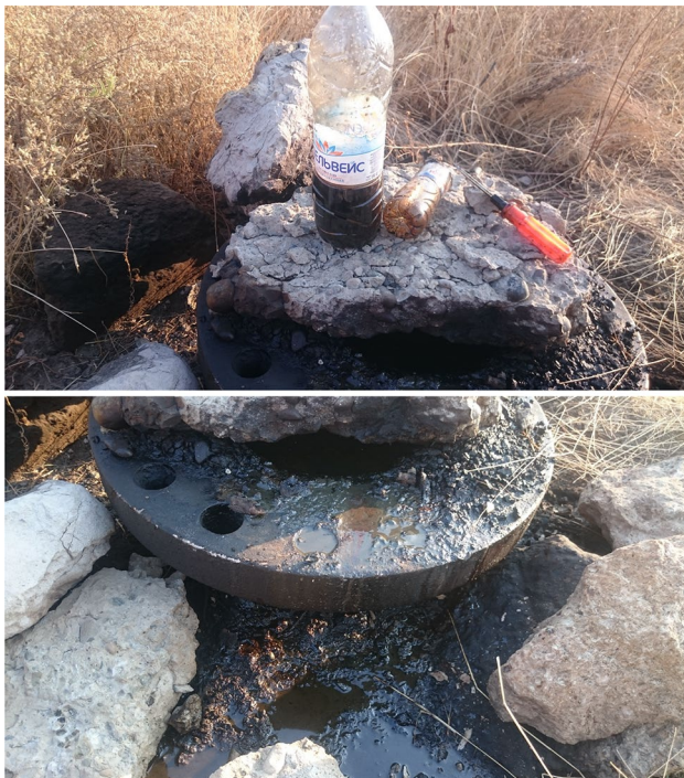
Fig. 5 Oil shows at the casing head of Well # 7 Selskaya
