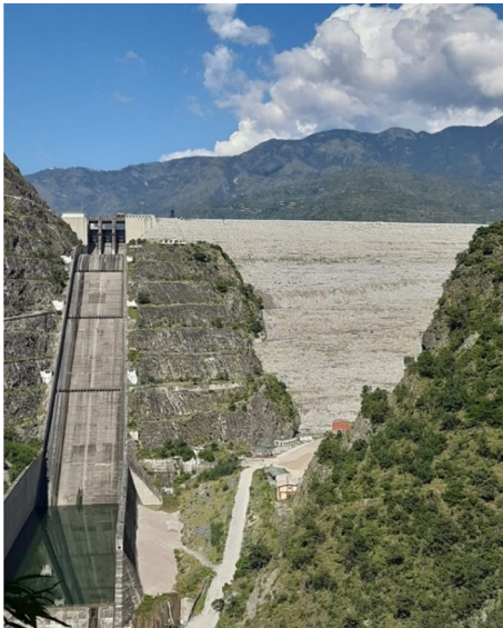
Fig. 2 Front View of Tehri Dam
