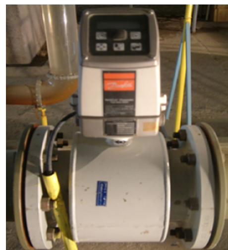
Fig. 6 Flowmeter installed in the model
