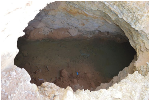
Fig. 12 Landslide in the gallery of the foggara of Mohamed Abdellah. (photo. Authors 2018)
