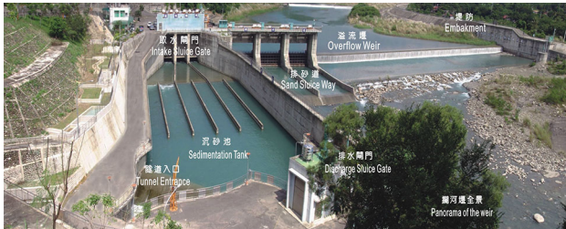
Fig. 3 Photograph of the Chiahsien Weir
