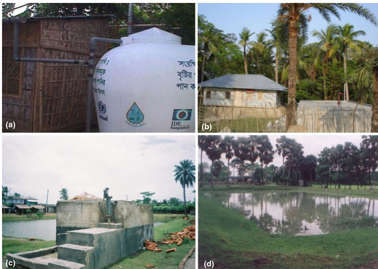
Fig. 1 Drinking water options: a household-based rainwater harvesting system; b community-based rainwater harvesting system; c PSF; d pond
