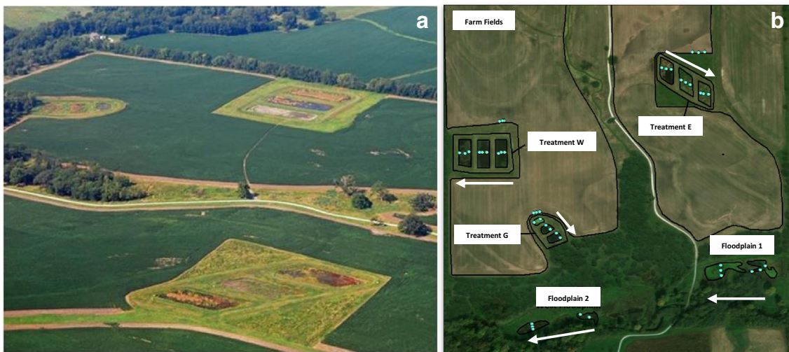
Fig. 1 a Aerial photo of the three wetland treatment areas constructed on Franklin Research and Demonstration Farm, Lexington, IL, and b) sampling locations in the wetland treatment areas, floodplains, and farm
