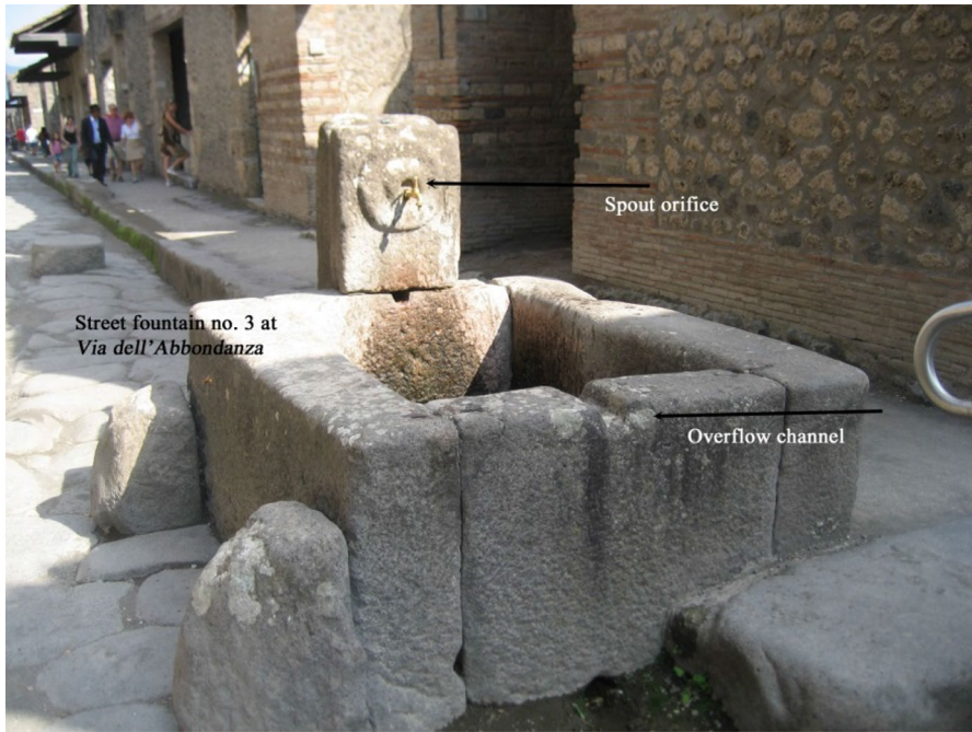
Fig. 3 Street fountain no. 3. The features measured by Moteleone et al. are indicated
