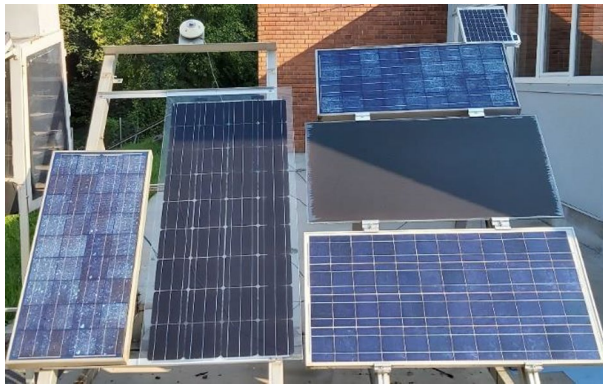
Fig. 4 Installation of PV modules
