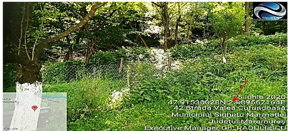
Fig. 9 Landslide located on Valea Cufundoasă Street, Sighetu Marmatiei Municipality (Source: GeoSES Project (Project GeoSES 2021))
