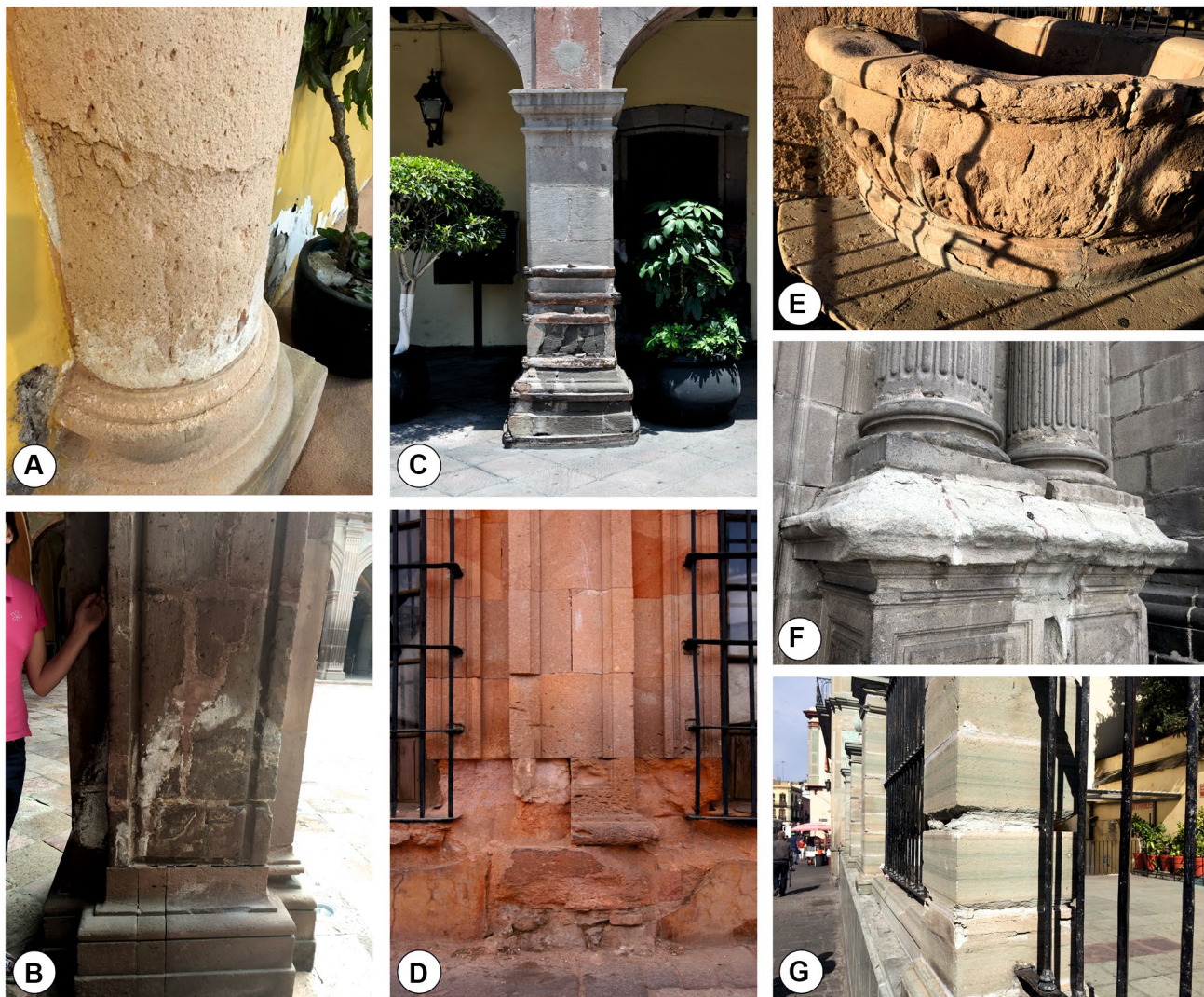
Fig. 2 Deterioration phenomena in volcanic tuffs. a Cantera Rosa de San Luis Potosí, b column of Escolásticas tuff with marked efflorescence of salt causing loss of material and discoloration, inner courtyard of the Faculty of Philosophy in Querétaro, c scaling and chipping with structural disintegration of a column from a building in the
