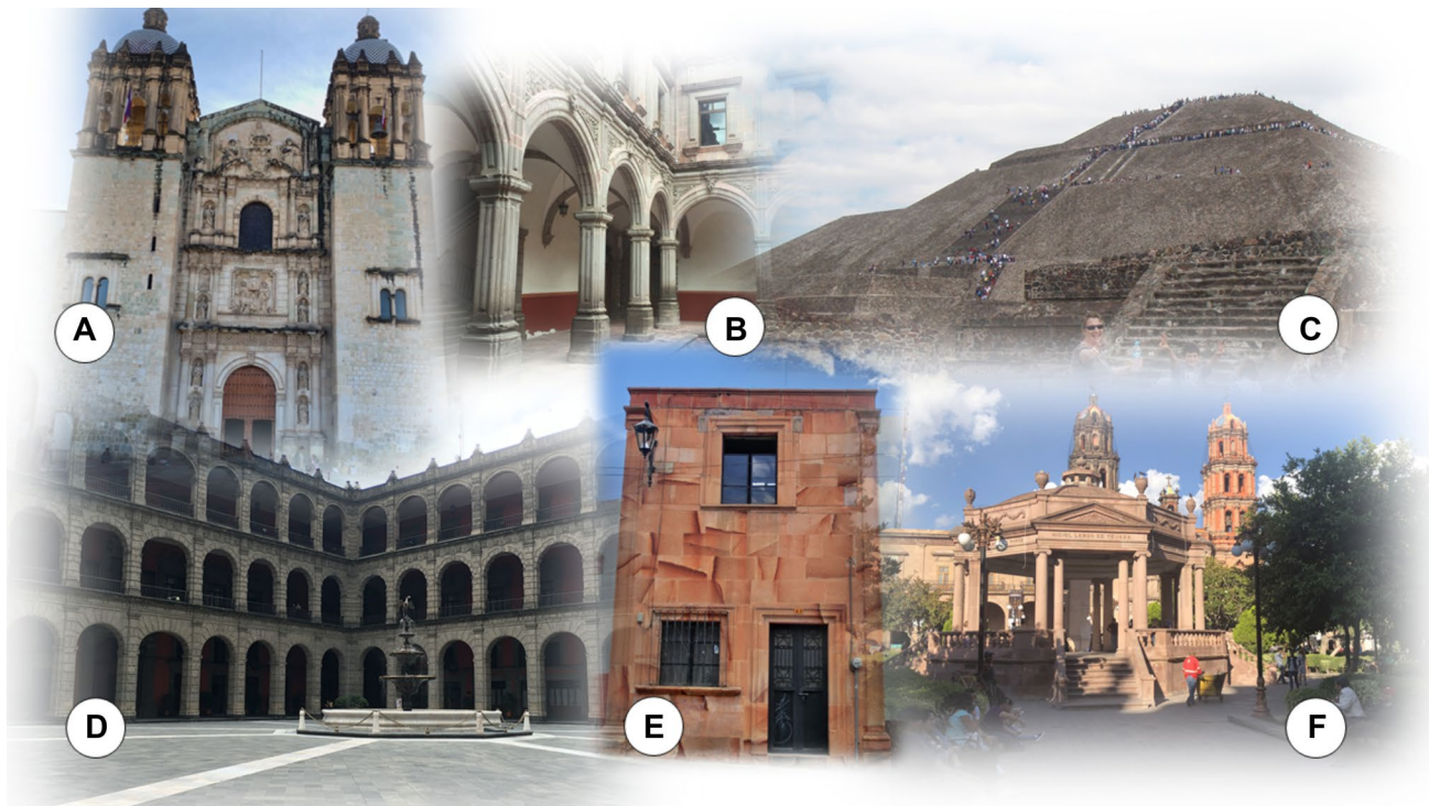
Fig. 1 Examples of different buildings and structures from the cultural heritage of Mexico built with volcanic stones. a Santo Domingo Temple, Oaxaca City (Cantera Verde tuff), b arches of the Faculty of Philosophy, Querétaro historical center (Escolásticas tuff), c Pyramid
