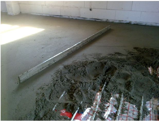
Fig. 1 Exemplary view of concrete floor screed during construction
