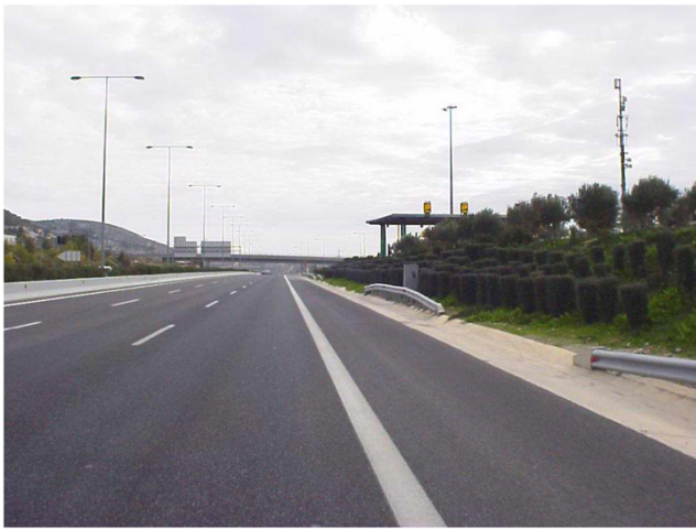
Fig. 2 Short break in guard rails
