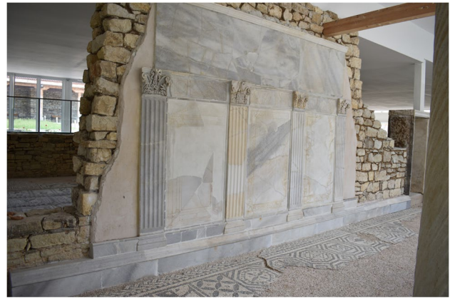
Fig. 2 Marble-plated wall with pilaster capitals at the Peristilium of the villa (Ph. V. Anevlavi, ÔAI/ÔAW)
