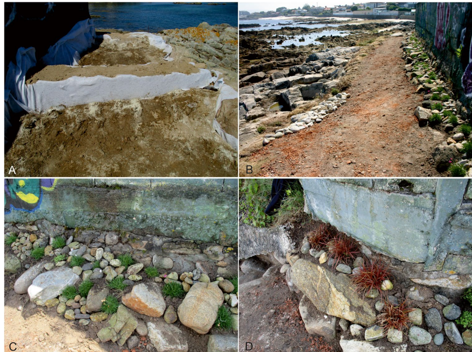
Fig. 23 A Construction of protective structures. (B) Final result after the conservation-restoration process. (C and D) Detail of the species Festuca glauca and Uncinia rubra used to stabilise the terrain
