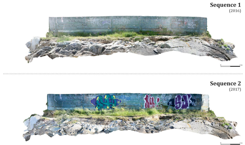
Fig. 18 Changes and anthropic aggressions suffered by the site, visible after the processing of both photogrammetric models. Frontal view of the models, from the north
