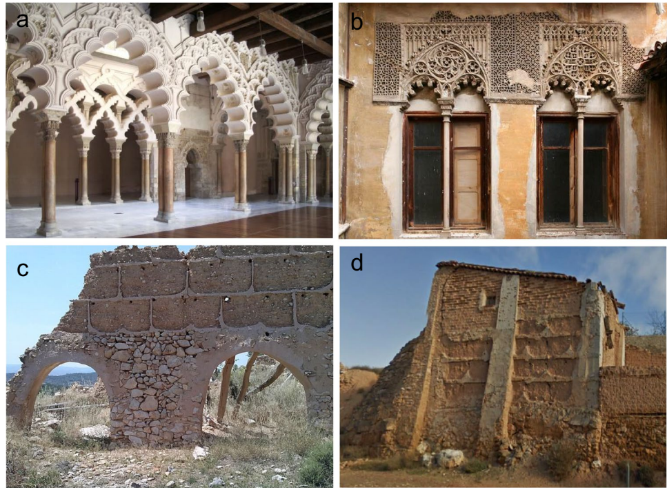
Fig. 1 Decorative and structural gypsum use: a decorative plasterwork, “Aljaferia” palace, eleventh century (Zaragoza, Zaragoza); b exterior plasterwork, “Los Luna” palace, fourteenth to sixteenth century (Daroca, Zaragoza); c arches built with gypsum stone masonry, rammed earth, and gypsum mortar (La Ginebrosa, Teruel), and d buttresses made of gypsum (Fuentes de Jiloca, Zaragoza)
