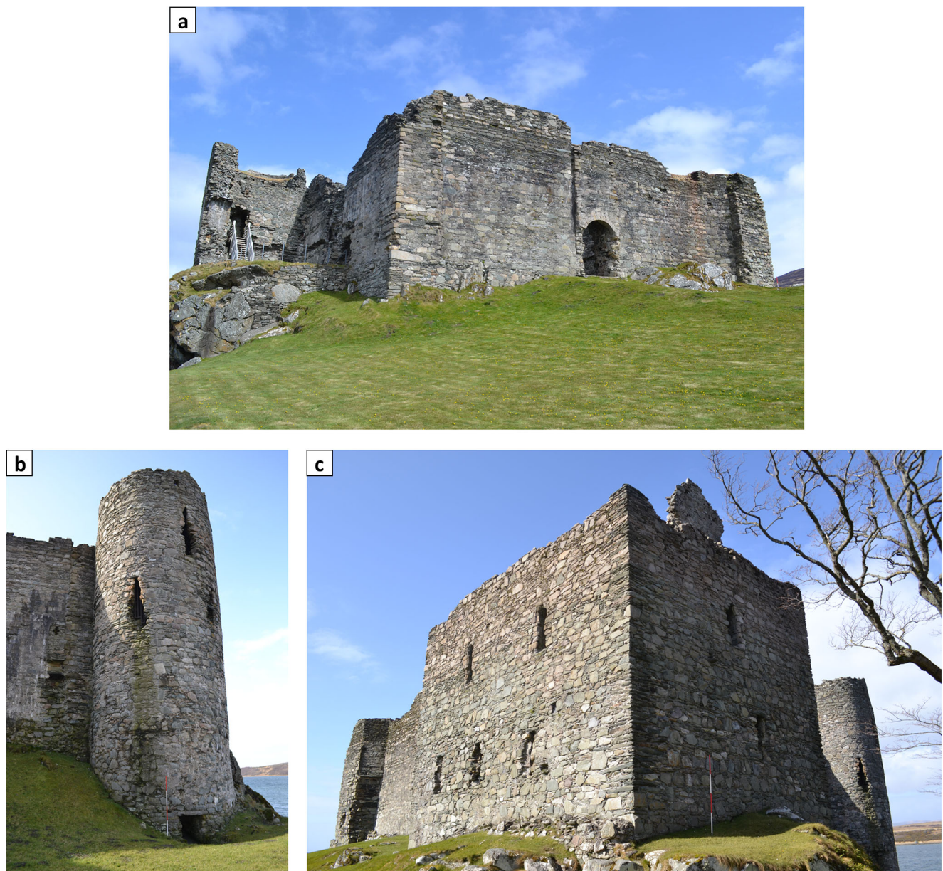
Fig. 4 a-c The main structural phases of Castle Sween. a Castle Sween from the southwest. Highlighting the sandstone-framed round arched main entrance and clasping buttresses of the primary phase enclosure; Romanesque features on which a c.1200 constructional date is based. The surviving upstanding sections of the otherwise collapsed secondary West Range and NW Tower are visible on the left of this image. No scale. b Castle Sween NW Tower from the north. Perceived architectural similarities between this circular garderobe tower and a feature at
