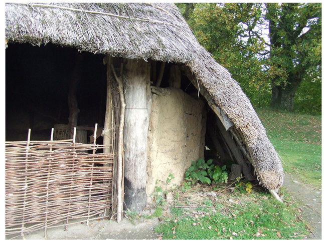
Fig. 11 Cookhouse Phase 4 rafters resting on the ground to east of doorway
