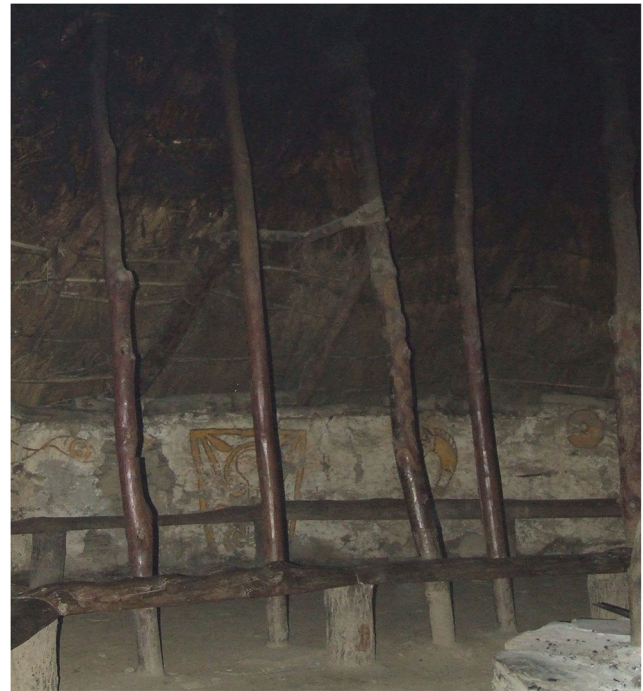
Fig. 24 Earthwatch roundhouse interior with benches round hearth set on the raised floor which has encased the rafter prop bases and hidden their stone pads, taken 2017
