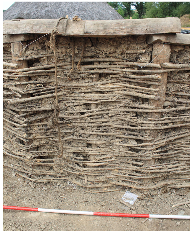
Fig. 25 Earthwatch roundhouse wattle wall exposed after the removal of the exterior daub
