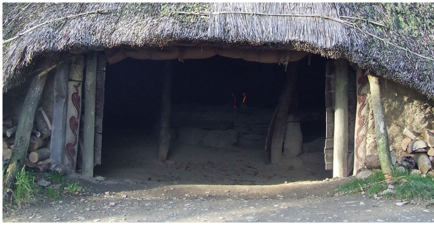
Fig. 27 Earthwatch roundhouse doorway modifications supporting the decorated original door jambs, taken 2017; note the naturally-formed eaves drip gully across the threshold
