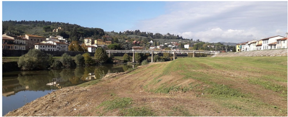
Fig. 5 Walkway, upstream view
