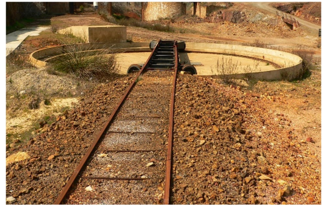
Fig. 13 Workshops turntable before restoration
