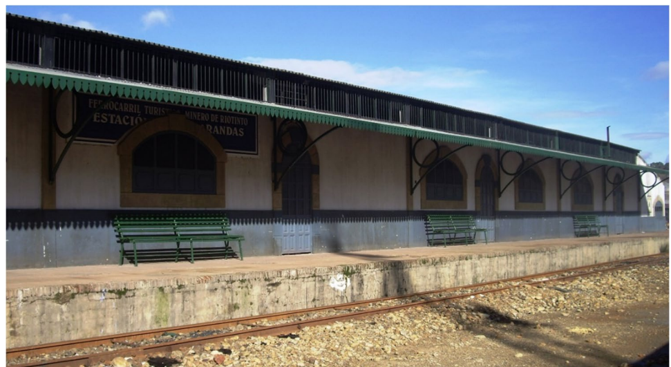
Fig. 9 Zarandas Station (present day)
