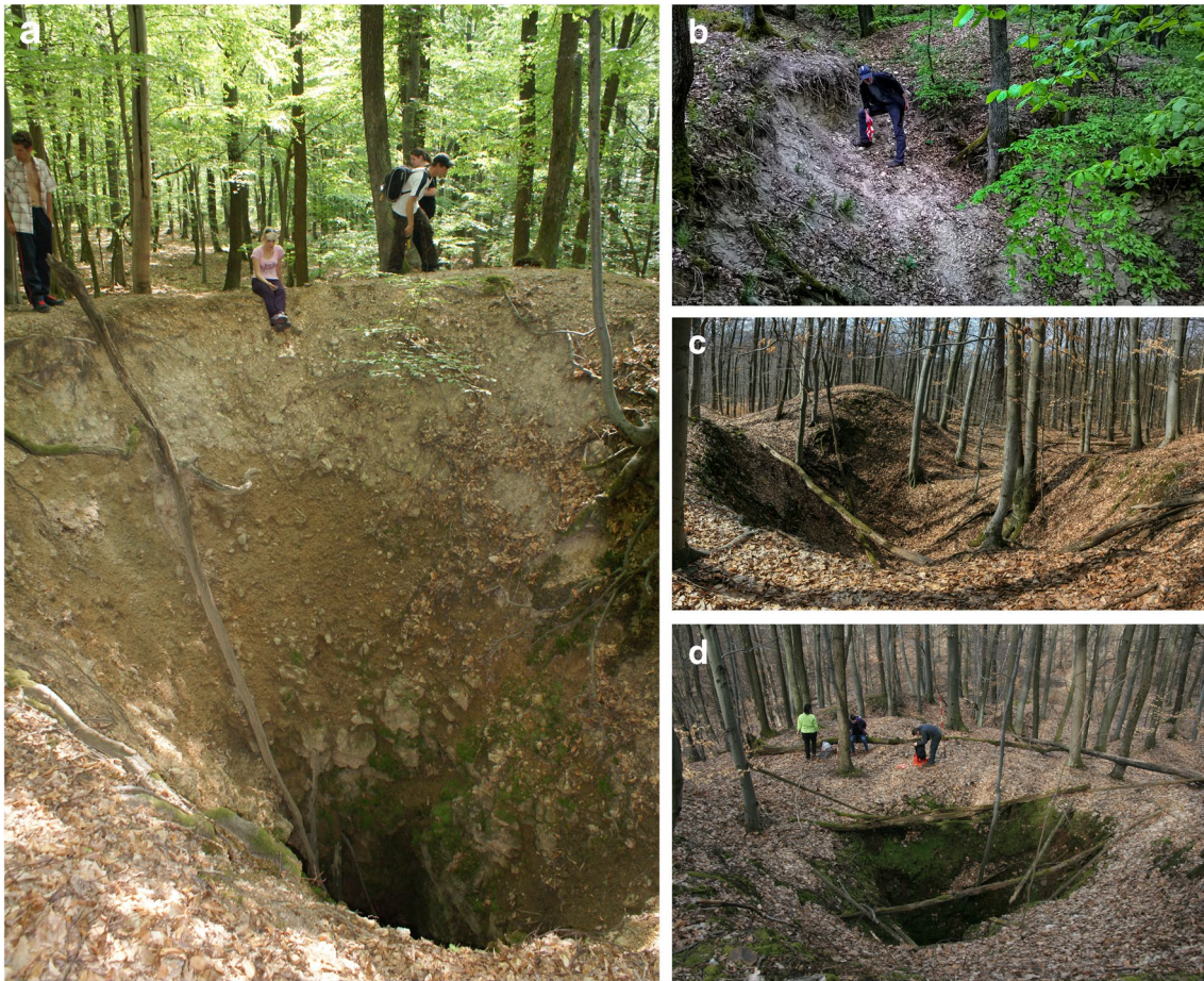
Fig. 7 Elements of the surface mining infrastructure. a A pit in almost original condition (not filled with waste) visible altered wall rock at the bottom, Joó Hill pitfield. b The rim of an average sized pit ( \downarrow 2 m, \varnothing 5 m, with mineral collector's reworking (white)). c Collapsed
