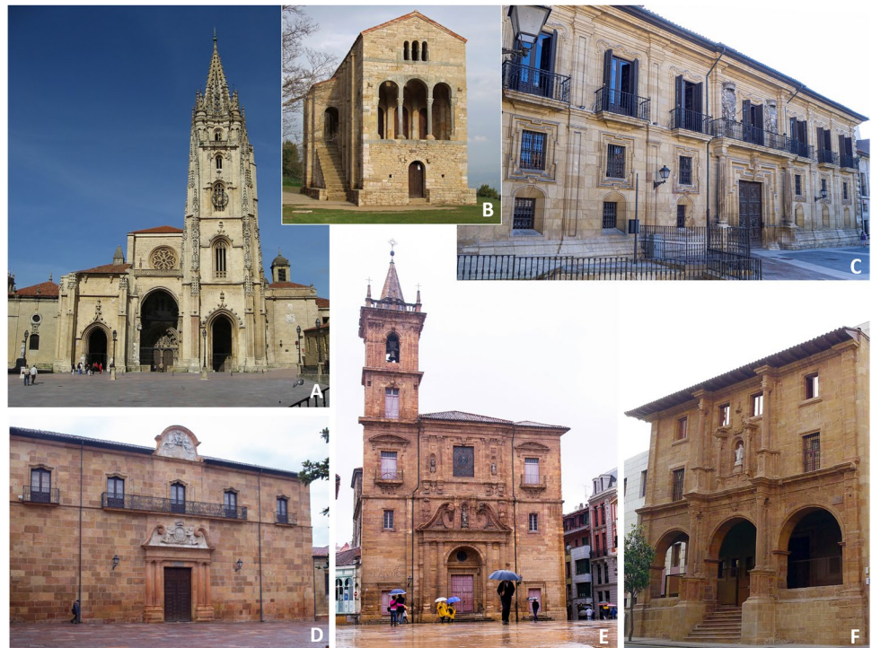
Fig. 2 Relevant monuments built with Cretaceous stone: Cathedral of San Salvador de Oviedo (A), Santa María del Naranco (B) and palace of Duque del Parque (C) with Piedramuelle lithotype. Facade of the cathedral cloister (D), church of San Isidoro (E) and convent of Santa Clara (F) with La Granda lithotype
