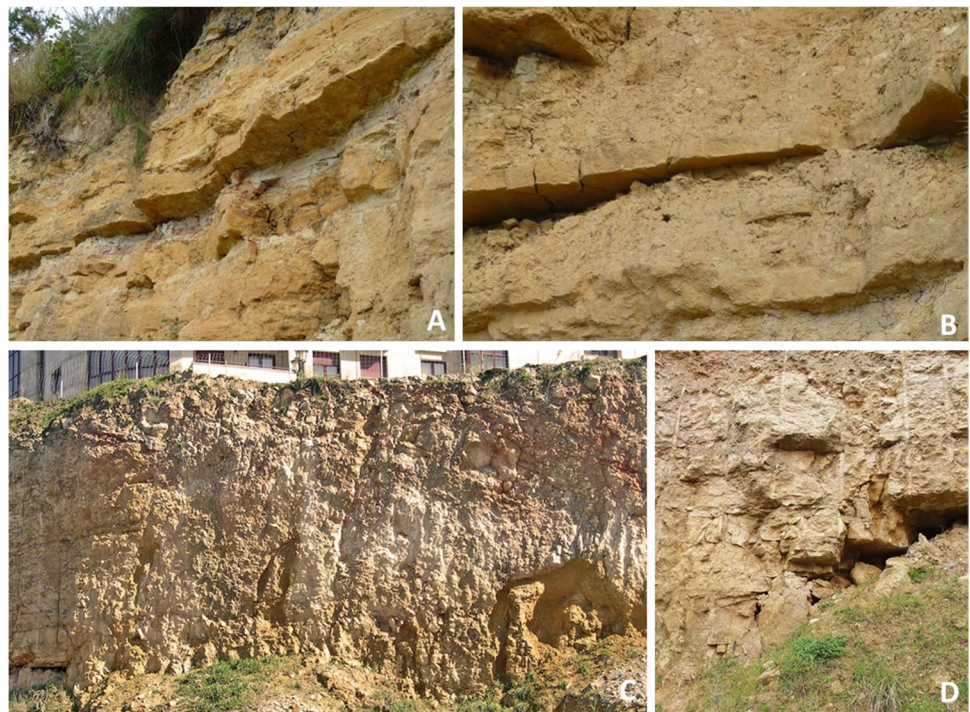
Fig. 9 Field appearance of the San Lázaro Formation in the old Santa Marina de Piedramuelle quarry (A and B) and the Oviedo Formations in the old Lavapiés quarry (C and D). See location in Fig. 3
