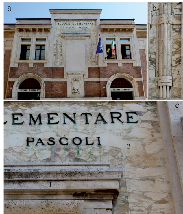
Fig. 4 Stop 2: the façade of the Pascoli School (a) with particulars of the Travertine slabs (b1 and c1) and of the brecciated marble from Carrara District (b2 and c2)
