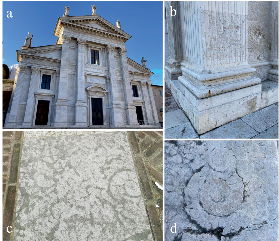
Fig. 9 Stop 6: the façade of the Cathedral mostly made of lithotypes of the Bugarone Group (a) characterised by degradation phenomena of detachment and staining due to pyrite oxidation (b); particulars of the square adjacent to the Cathedral, paved with bricks and blocks of the Bugarone Group characterised by big fossils of Ammonites (c, d)
