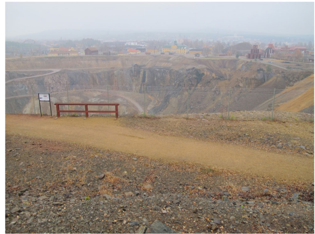
Fig. 1 The location of Falun Mine and the central part of the UNESCO World Heritage Great Copper Mountain in Falun. The view is to the east and shows the “Great Pit”, which is a remnant from a mine collapse in 1687 and the later expansion of the mine up until the twentieth century. In the background are older buildings of various ages from the mining activity from the seventeenth century to the twentieth century, where there is also a local museum and a World Heritage centre. (Photo: Magnus Hellqvist)
