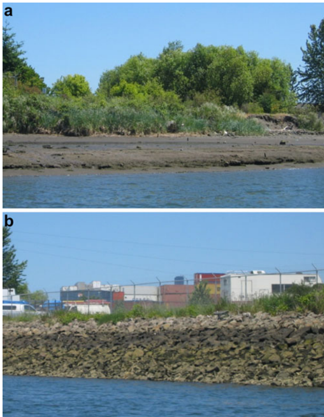
Fig. 2 Photos of a typical a unarmored and b armored study site at low tide
