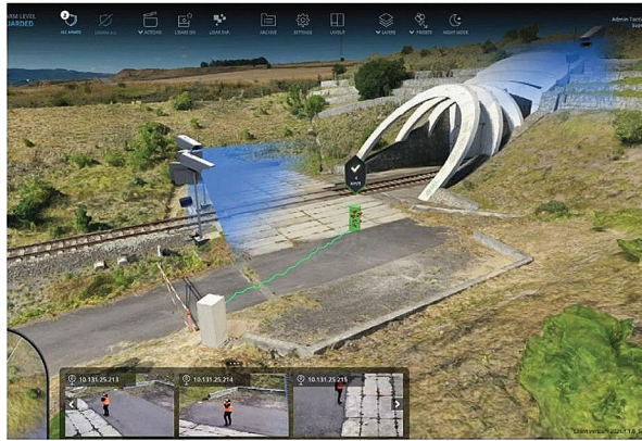
Fig. 10 View of the Břežno tunnel portal through the Accur8vision visualization software - the person in the detection zone is displayed both graphically and visually using a rotating camera tracking his/her movement (Hexagon 2023a)
