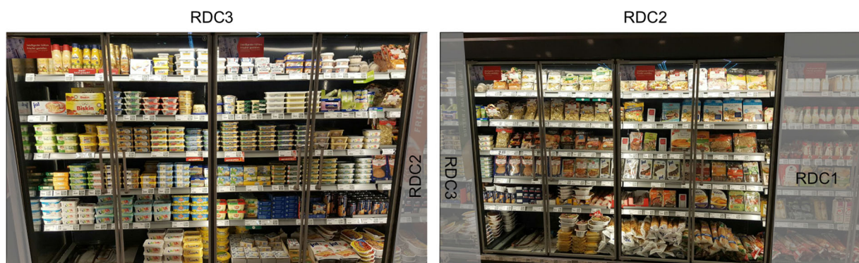
Fig. 1 Photos from the investigated supermarket, showing the neighbouring refrigerated display cabinets, RDC_2 and RDC_3
