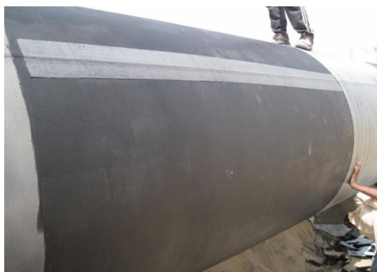
Fig. 8: Geotextile mesh backed tape applied on large diameter water pipeline
