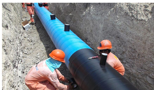
Fig. 7: Field cold applied viscoelastic tape: inner layer (blue), outer layer (black) (Color figure online)
