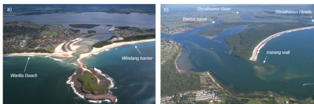
Fig. 8 (a) The entrance to Lake Illawarra in 2001 at the commencement of construction of a training wall on its southern margin. At this time sand from Warilla Beach could be moved into the lake entrance. This has since been prevented by the training wall, and Warilla Beach has been nourished with sand from the channel. (b) The mouth of the Shoalhaven River with Crookhaven Heads in the foreground. Berrys Canal is continuing to widen
