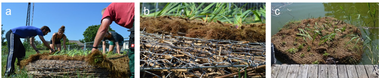
Fig. 1 Installation of first floating wetlands. (A) Pre-cultivated coir mats with macrophytes were placed on the buoyant structure. (B) The carrier consists of an enveloping stainless steel net filled with native dry reed stems. (C) Installation was carried out from a jetty
