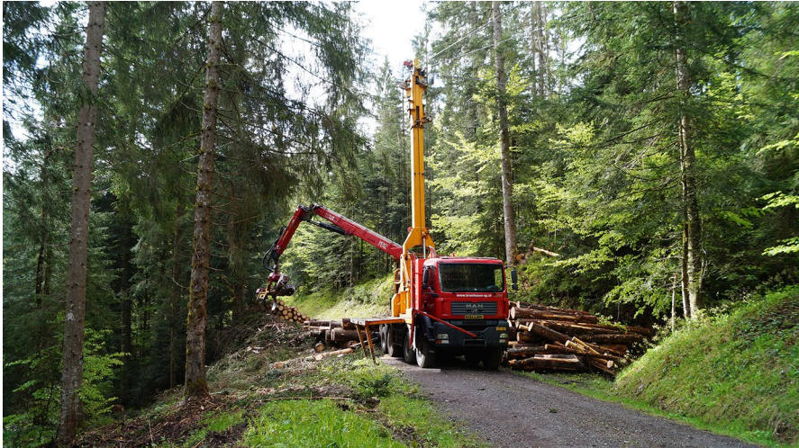
Fig. 2 The K507 is mounted on a truck and applied with a three-cable system due to the horizontal yarding direction. An Eckoboost (Koller Forsttechnik GmbH, Austria) was used as carriage, with a maximum load capacity of 4 t (Fig. 3)
