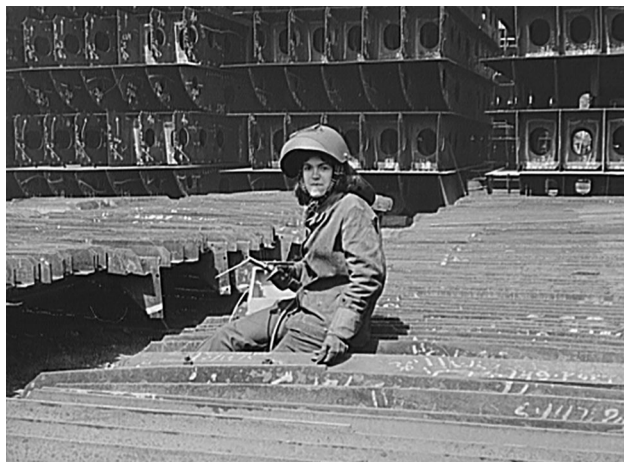
Fig. 2. An unidentified “Wendy the Welder” at the Bethlehem-Fairfield Shipyard, likely butt welding the vertical joints from Ref. 2. Original photo: Library of Congress (Arthur S. Siegel, photographer, U.S. Farm Security Administration).
