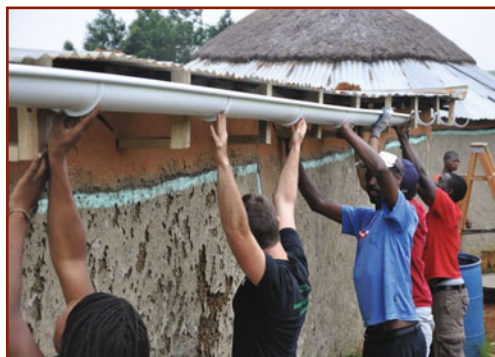
Kettering students work with Vukuzenzele community members to construct rainwater collection systems.
