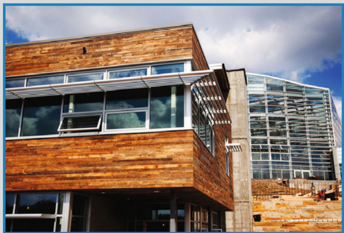
The Center for Sustainable Landscapes exterior, clad in siding made from repurposed barn wood. (Photo credit: Alexander Denmark Photography.)
