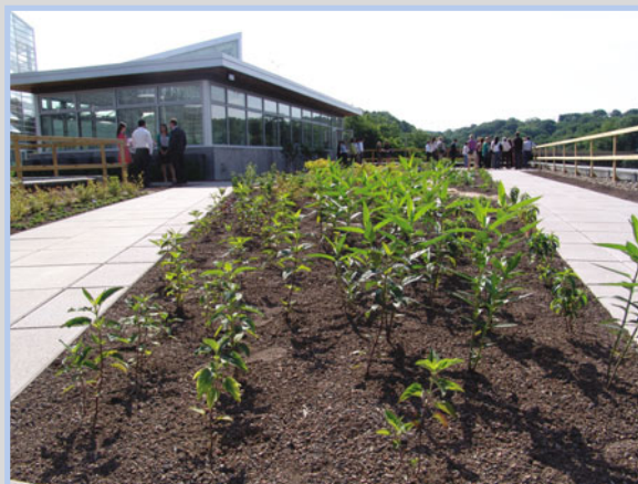
Figure 6. A “green roof” on the CSL reduces stormwater runoff, while also helping to insulate the building.
