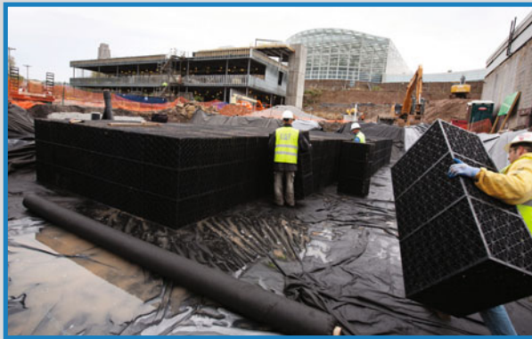
Figure 10. Aqua-Blox™ cubes buried underground within an impermeable basin capture rainwater that will be used for watering Conservatory plants. (Photo credit: Alexander Denmarsh Photography.)
