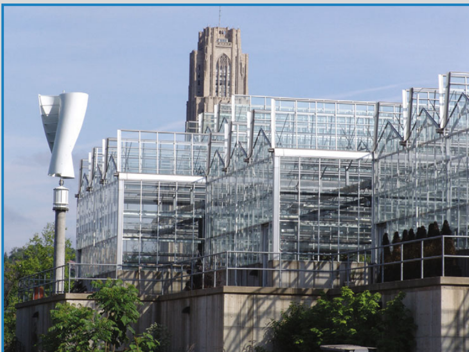
Figure 8. This vertical axis wind turbine is expected to generate 50 percent more electricity annually than traditional propeller models under similar conditions, and is safe for urban use. Also pictured in the photo are Phipps' production greenhouses (foreground) and the University of Pittsburgh's Cathedral of Learning.
