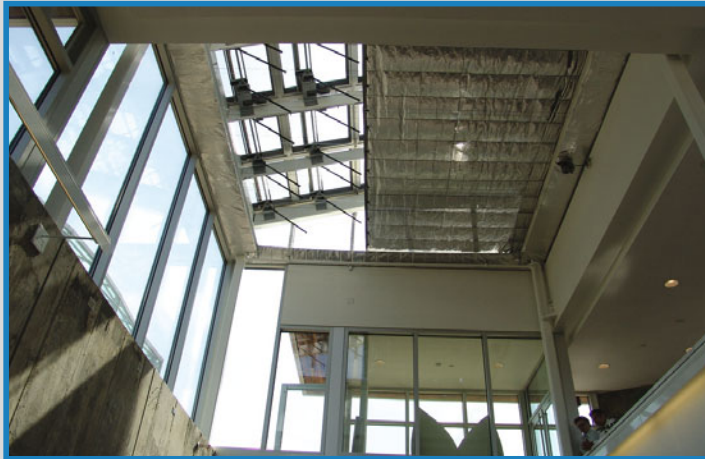
Figure 9. The centerpiece of the CSL is a striking atrium that is 100% passively cooled. Passive heating strategies and winter solar collection take advantage of thermal massing in the walls. Capturing available natural light is another design priority of the building, minimizing the need for electric illumination.
