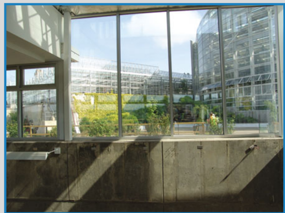
Figure 9. The centerpiece of the CSL is a striking atrium that is 100% passively cooled. Passive heating strategies and winter solar collection take advantage of thermal massing in the walls. Capturing available natural light is another design priority of the building, minimizing the need for electric illumination.
