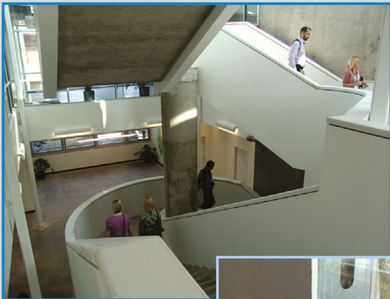
Figure 9. The centerpiece of the CSL is a striking atrium that is 100% passively cooled. Passive heating strategies and winter solar collection take advantage of thermal massing in the walls. Capturing available natural light is another design priority of the building, minimizing the need for electric illumination.
