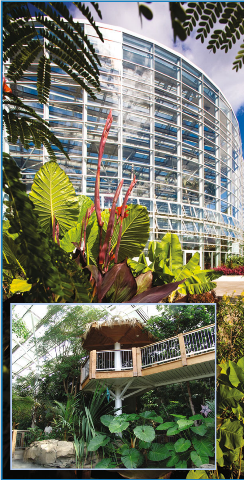
Figure 4. (Top): Phipps hit upon an unconventional building shape for its Tropical Forest Conservatory that permitted the use of insulated roof glass, while still maintaining light levels for growing plants. (Inset): Another radical change to conservatory design at the Tropical Forest is allowing half of the roof vents to be opened. This, combined with earth tube cooling and other innovations, has enabled the structure to be 100 percent passively cooled—essentially eliminating the “greenhouse effect” of the greenhouse.
