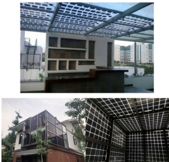
Fig. 10 Photographs of BIPV shading application and BPV applied as window shading devices.
