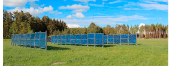
Fig. 8 Vertically mounted bifacial APV system in Sweden (adapted from Ref. [60] under the terms of CC BY license).
