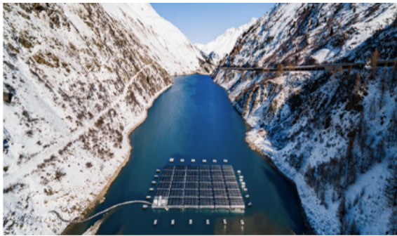
Fig. 14 448 kWp FPV at an altitude of 1800 m in Lac des Toules (adapted from Ref. [109] under the terms of CC BY license).
